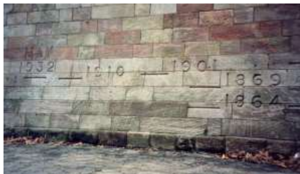
Flood marks recorded on Trent Bridge, Nottingham
