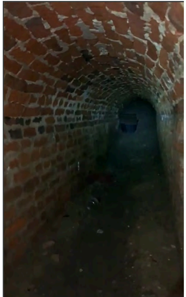
Exhibit A: the tunnel
