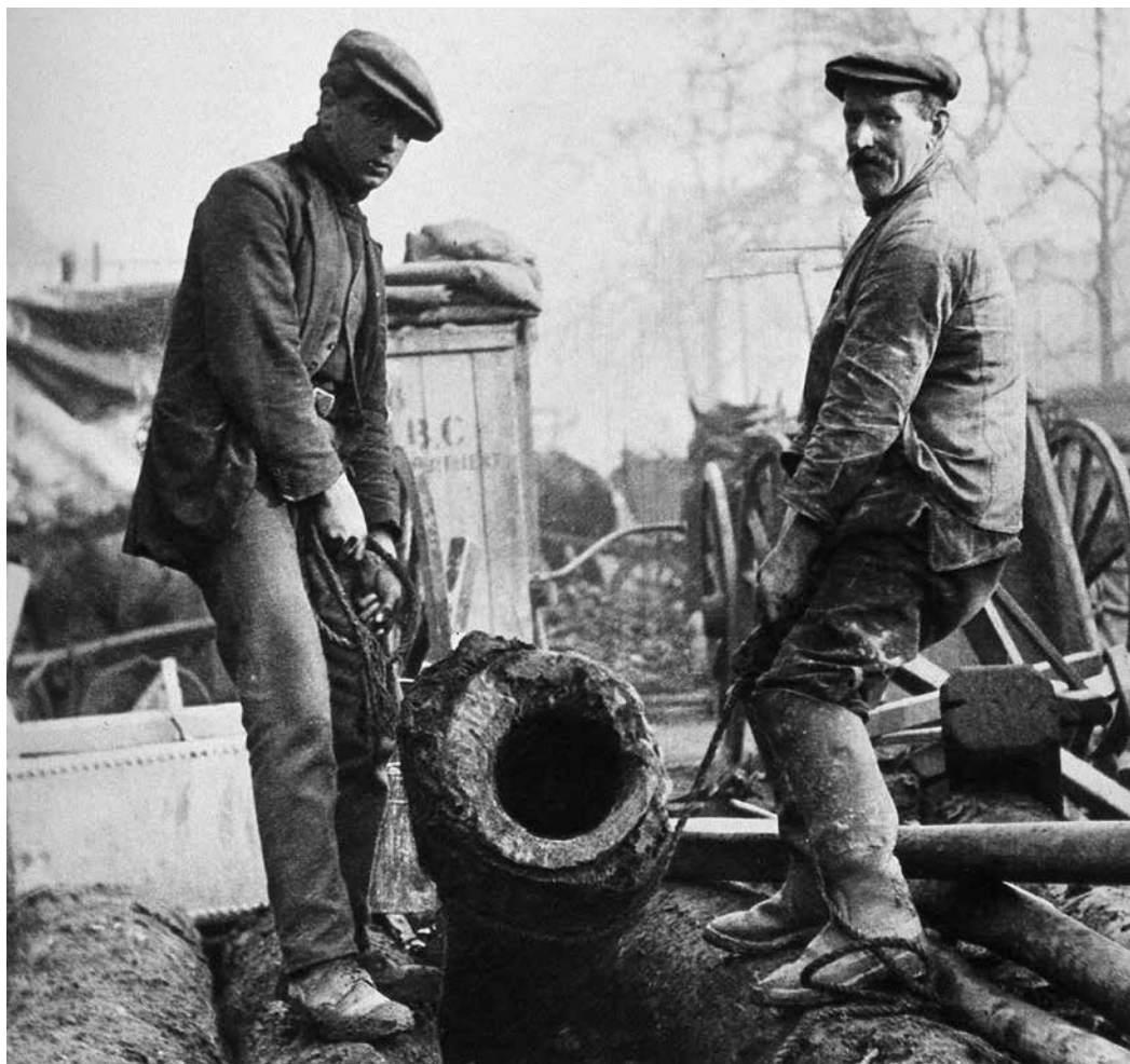
Elmwood water pipes uncovered in London, dating from the 17th century. (Wellcome Collection)
